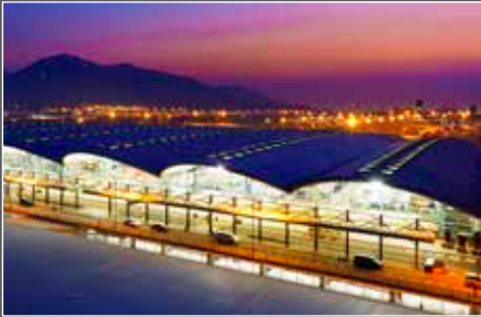
Hong Kong International Airport
